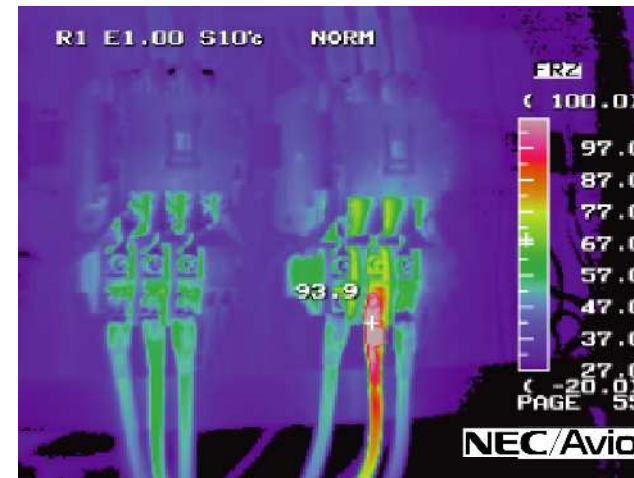
Short-circuit in switch board
